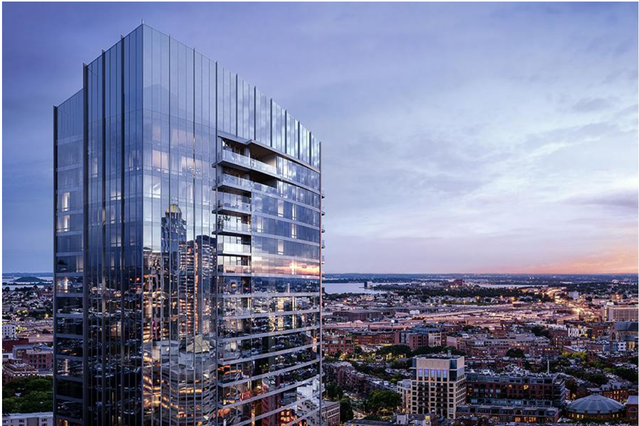
A rendering of the exterior of Raffles Boston by The Architectural Team / Image by Binyan Studios
